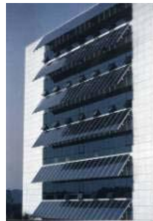
Figure 40: Solar panels on the facade of an office building, Image obtained from Eastside casestudy
