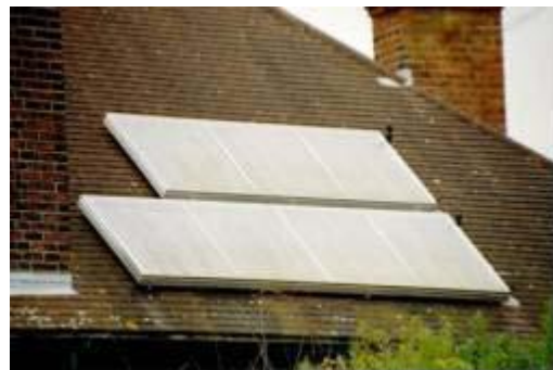
Figure 37: Picture of a flat panel collector. Obtained from the Birmingham Case Study
